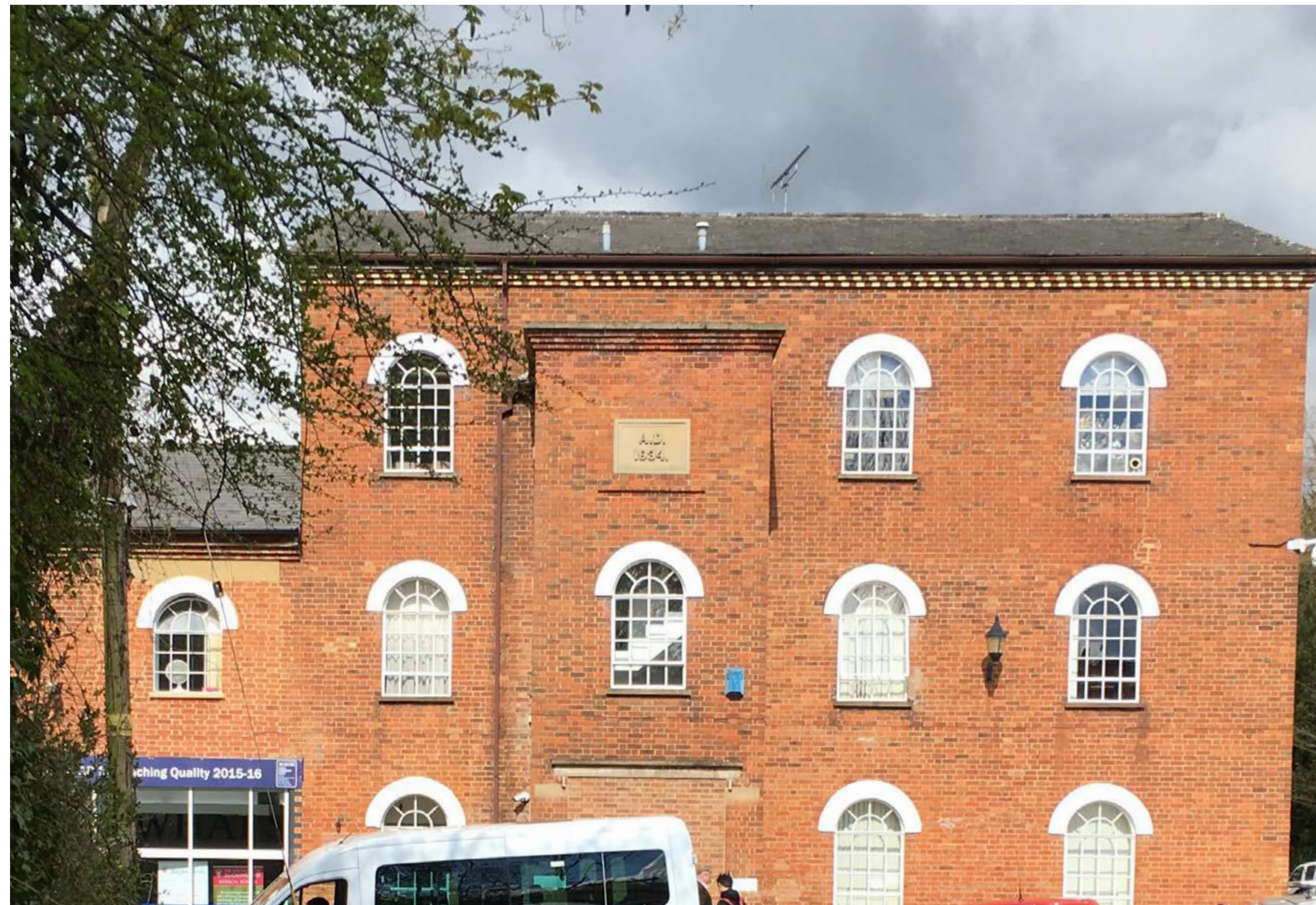
The Chandos Road Building - Mixed Orange Brick with White Painted Window Headers and Metal Multipaned Windows
