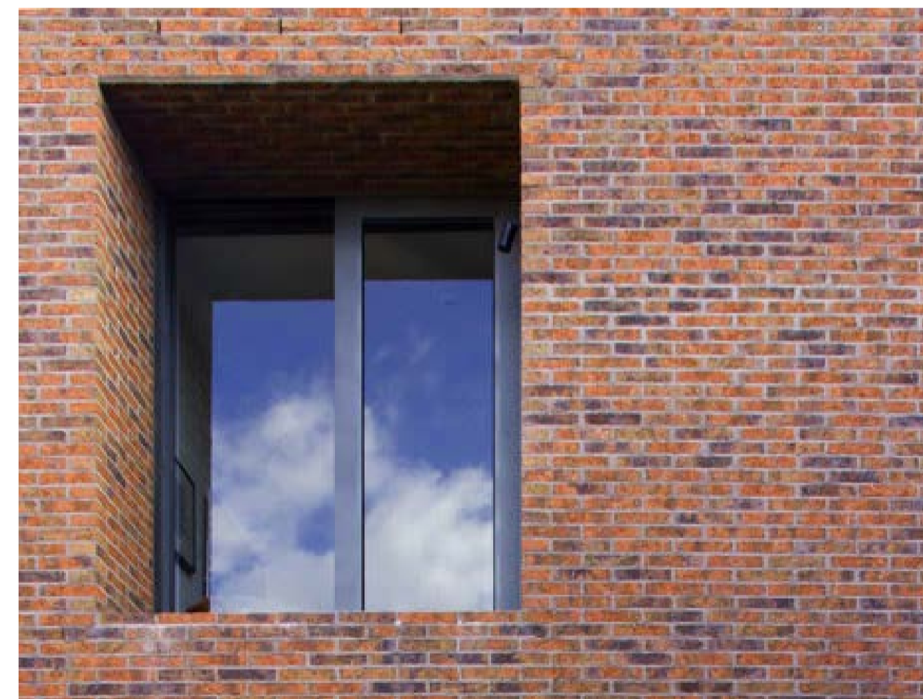
Mixed Red/Orange Brick for the Main Walls of the Building
