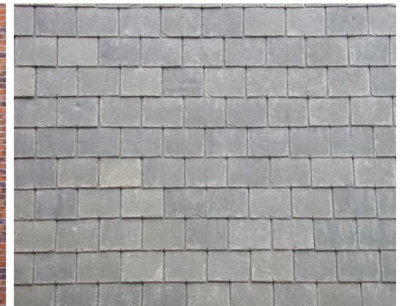
Natural Slate Roof
